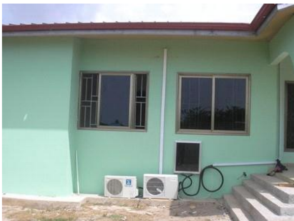
Our Solar AC used in Africa office
