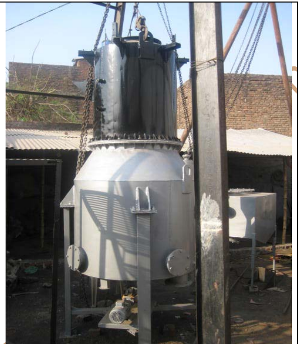
Gasifier under assembling
